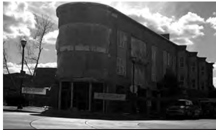
TIGARD APTS • 166 UNITS SW ASH & BURNHAM STREET TIGARD (under construction)
