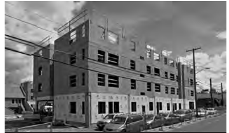
13 WEST APTS • 92 UNITS 1314 SW COLUMBIA STREET VANCOUVER (under construction)
