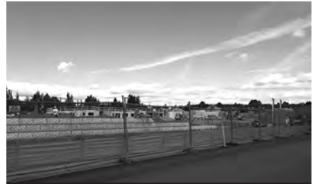
SCHOLLS APTS • 240 UNITS SW 135TH & SCHOLLS FERRY BEAVERTON (under construction)
