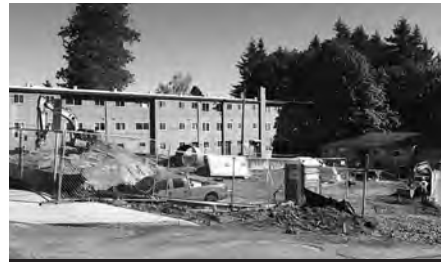
OHSU APTS • 12 UNITS 956 SW GAINES STREET SW PORTLAND (under construction)
