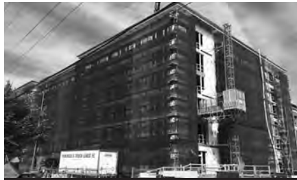
TAYLOR APTS • 121 UNITS 1551 SW TAYLOR STREET SW PORTLAND (under construction)
