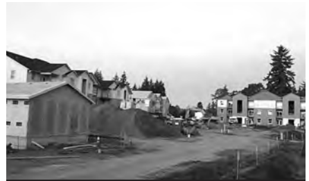
WEBSTER RD APTS • 120 UNITS 18121 WEBSTER ROAD GLADSTONE (under construction)
