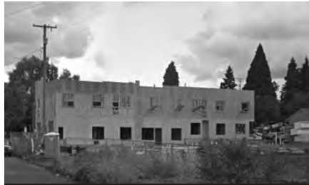
VVII • 48 UNITS 505 E 15TH STREET VANCOUVER (under construction)
